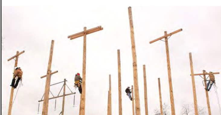
Students practice working on powerline equipment in Tri-County Career Center's Powerline Technology Program. The program helps students land good-paying jobs after high school.
