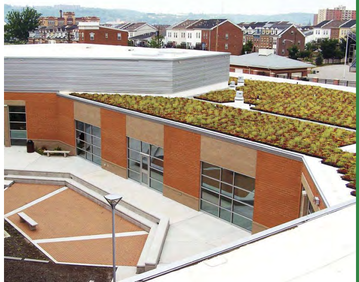
Taft High School's 33,000-square-foot green roof was funded by a grant from the Cincinnati Metropolitan Sewer District.
